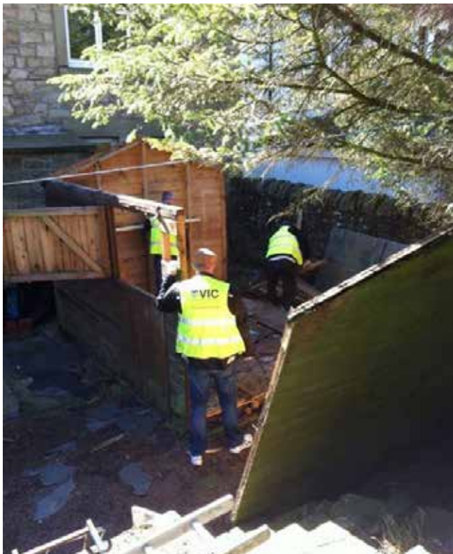
Dismantling a shed for an elderly veteran in Haslingden
