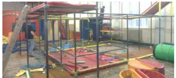
Dismantling a children's play for High Level in Rochdale
