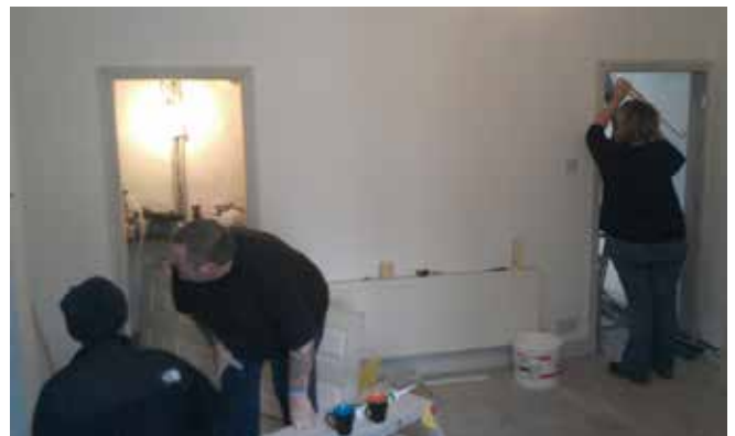
Renovating a house for a young family affected by cancer
